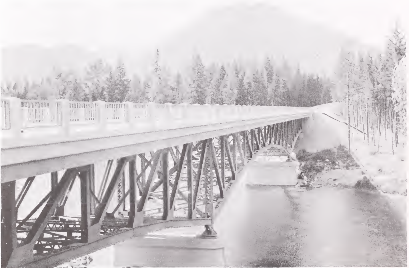
The West Glacier Bridge (Photograph courtesy of John Morrison).
